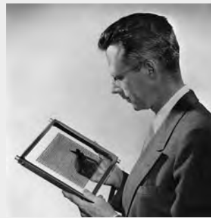
Coincident Coil Magnetic Core Memory: Jay holding a 64 \times 64 core memory plane, 1954. Picture used with the permission of The MITRE Corporation. Copyright © The MITRE Corporation. All Rights Reserved.
